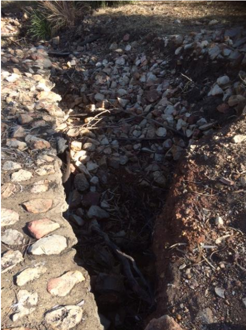
Scouring at Nindigully Weir
