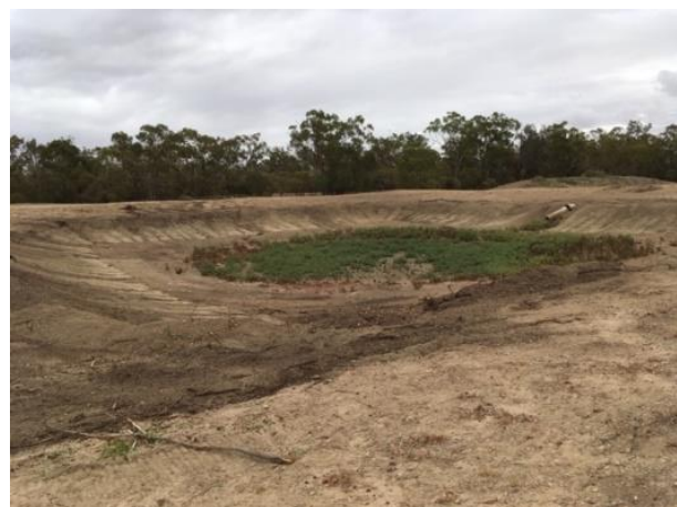
Photos Above: start of works at Boomerang dam – clearing dam edge then centre desilting and placement of bentonite, repair drainage.
