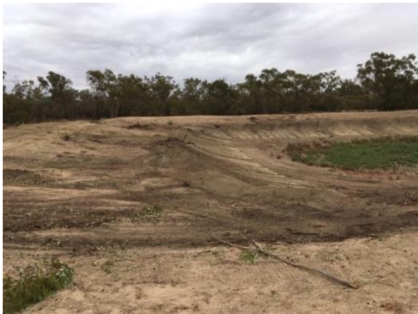
Photos Above: start of works at Boomerang dam – clearing dam edge then centre desilting and placement of bentonite, repair drainage.
