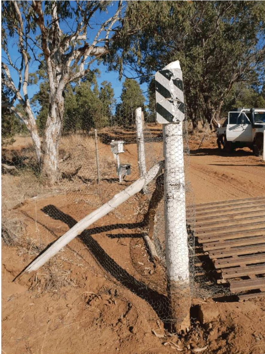
Replaced stay rail on the Cornwall Grid assembly
