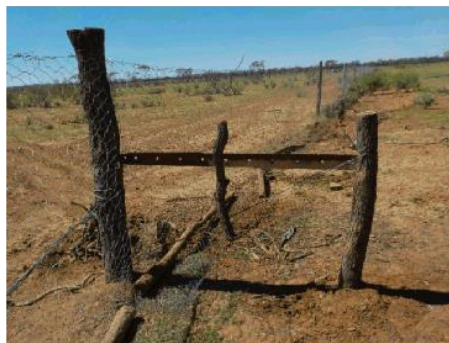
Replacing corner stay assemblies
