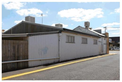
VIEW OF BUILDING FROM EAST IN LANEWAY SHOWING DIFFERENT STAGES OF CONSTRUCTION AND CLADDING DAMAGE AT BASE
