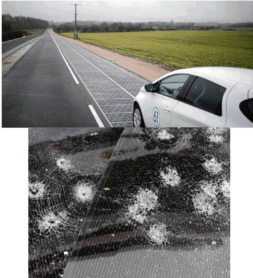
Figure 78: Normandy France 1 km solar road at start-up and problems experienced with damage
