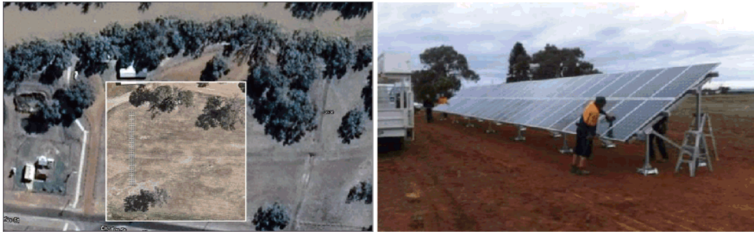
Figure 25: WTP showing "traditional" ground mounted system that can have a high GCR when installed in a single line of two panels wide.
