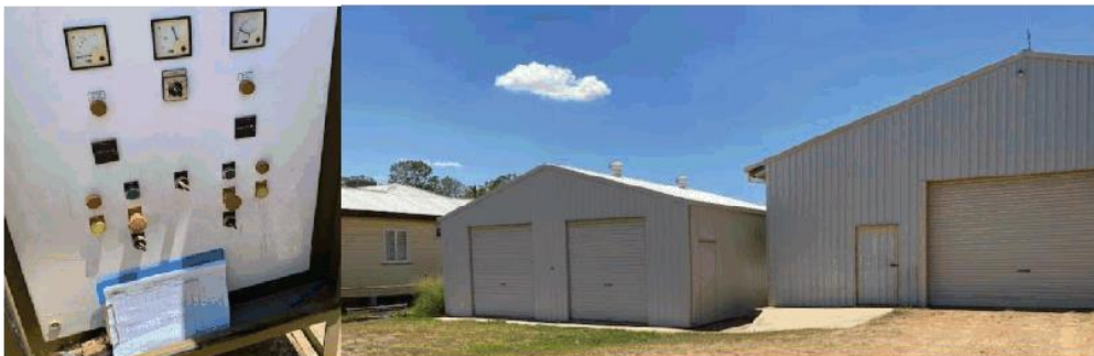
Figure 15: St George Pump Station 2. Image on the right shows shed suited to roof mounted PV solar. Largest loads of the sewer pumps at 20,195kWh pa, requiring ~11.3 kWp for energy neutrality.
