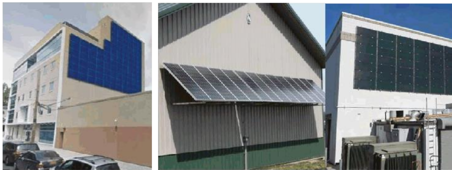
Figure 32: Example vertical installation of solar panels
