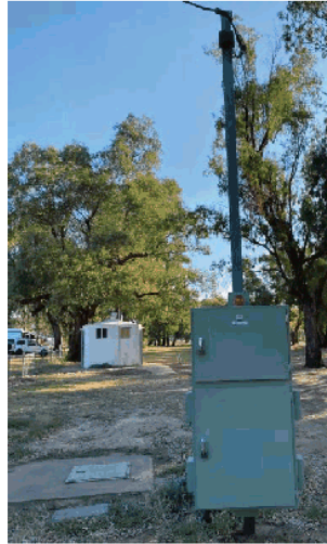
Figure 19: St George Pump Station 6. This location is less suited to a ground mounted system due to the openness of the location and utility as parklands near the river; hence there may be an opportunity for power to be reticulated from an array at #3 or to collaborate with the adjacent caravan park.
