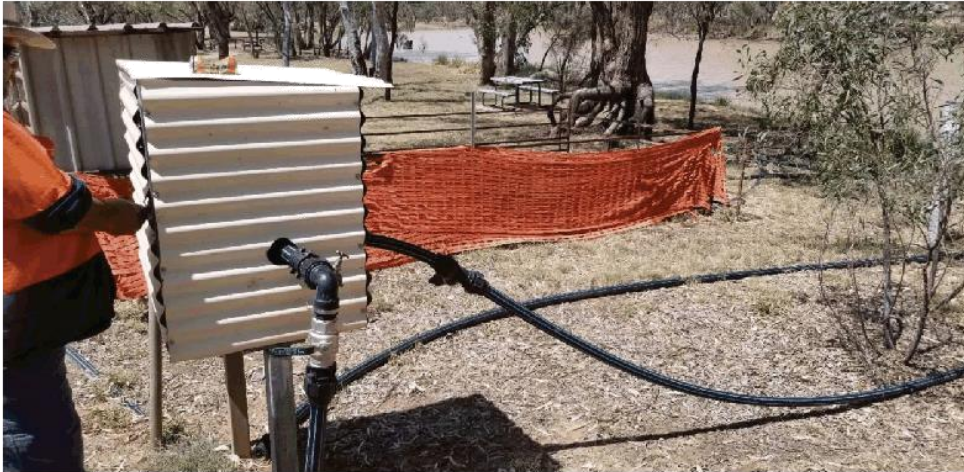
Figure 54: 1.4 kW pump on bank of Moonie River, Nindigully.
