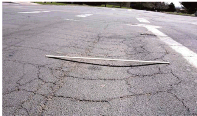
Figure 92: Rutting in a road
