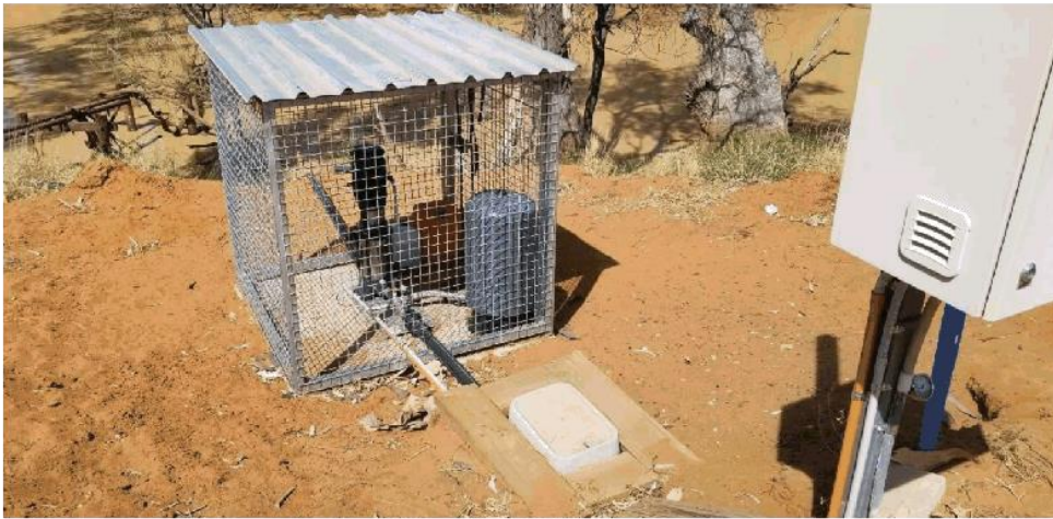
Figure 50: 3.0 kW river water pump
